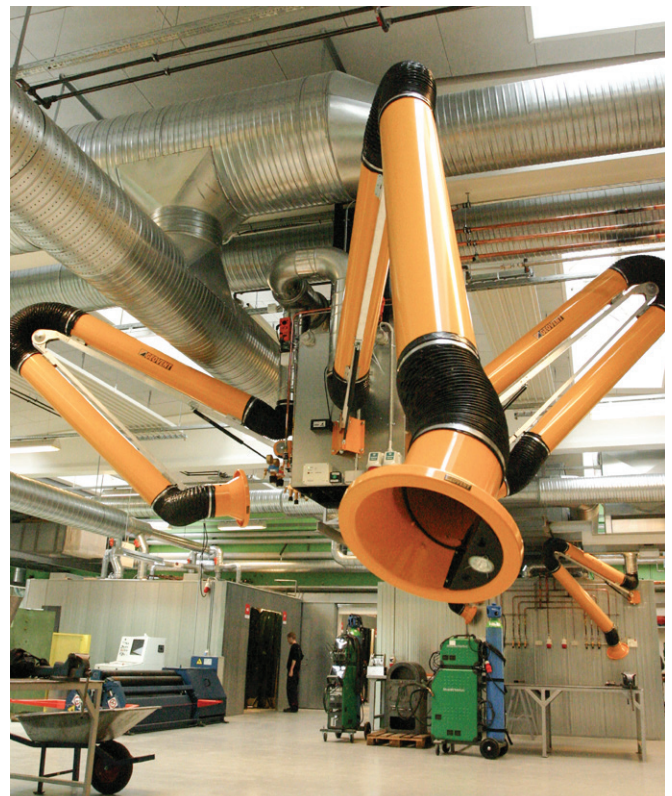
Complete construction of technical school with welding cabins and welding station.
