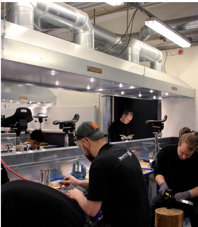
Extraction Hood at a school
