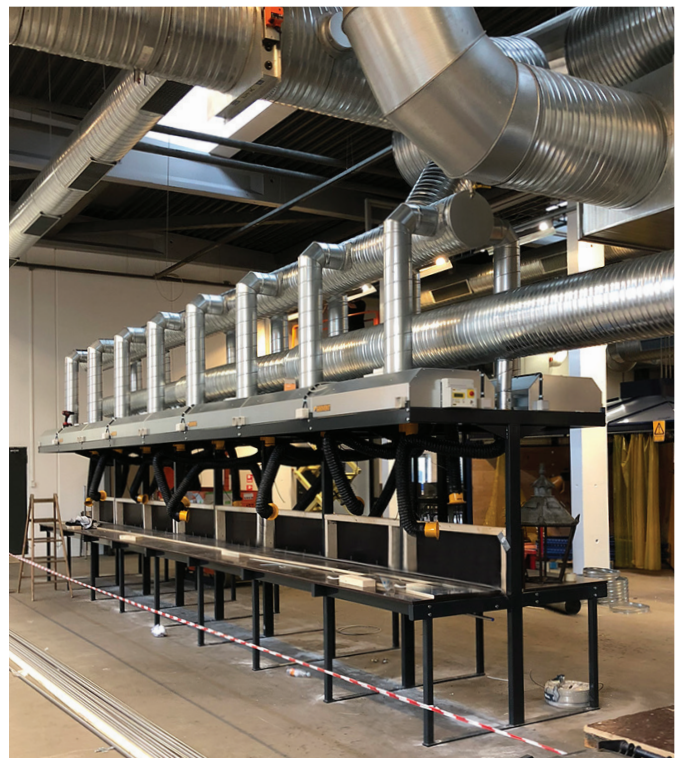
As seen in the picture, the hoods can be mounted in series so that the length of the hood itself can almost become infinite.
