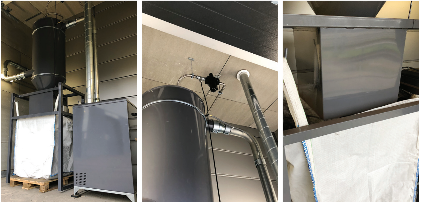
HVU Solo. Stand-alone side channel blower module.
