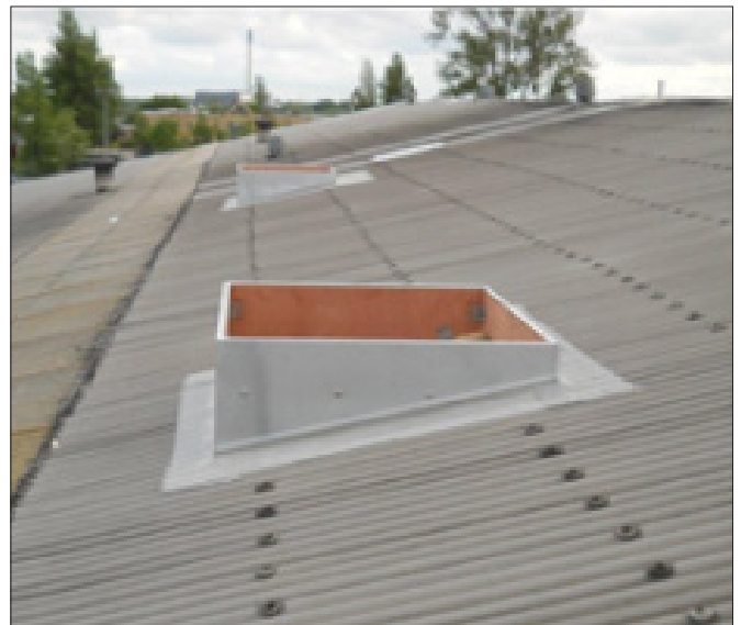
Example of base on sloping roof
